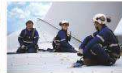
Service technicians at a V150-4.3MW turbine
